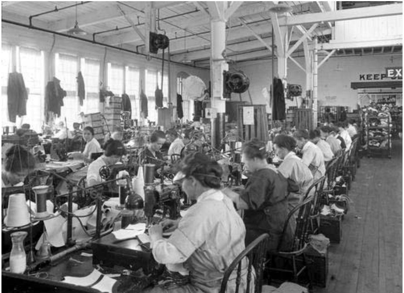
Figure B-30: Sewing uppers together, Endicott-Johnson Company, Endicott, 1917 (from NYS Archives )
