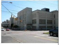
Massive 3-story rectilinear concrete clad steel framed industrial building. Features several full-height projecting pavilions, some with molded old-styled IBM globe logo. Many windows feature frosted glass block with hopper windows inserted into original large window openings. Some openings infilled. Saw-tooth detail at parapet of roof; large penthouses on roof. Raised skyway connects
