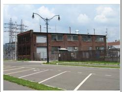
2-story rectilinear steel framed brick-clad industrial building with flat roof. Primary west elevation features large multi-pane metal industrial windows with raked sill. Other elevations retain many of the original rectangular metal industrial windows with small concrete sills set between shallow brick pilasters. On same parcel as 366 Water St (B).
