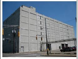
6-story rectangular reinforced concrete industrial building. The majority of windows have been infilled, although the structural framework of building is intact; some sills and spandrels are still visible. Some loading docks installed on ground level.
