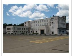
4-story rectilinear industrial building; first 2 stories constructed of poured in place concrete, upper stories added later to east half of building constructed with stuccoed brick. Flat roof with slightly shaped parapet and five-story corner stair tower. Some 8/8 metal sash windows, many infilled windows. Features loading bays on south elevation, 1-story portion on east and connected one-story building once used as an Endicott-Johnson leather storage warehouse.
