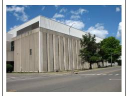
Large rectangular approximately 3-story Brutalist industrial building. Features molded concrete skin with vertical ribbing. One bay at eastern end of primary south elevation contains an entry door with a vertical glazed wall unit. Set between some concrete ribs are vents. Surmounted with 1-story unit clad with vertically-oriented corrugated metal sheathing. Now shares a large tax parcel with 1701 North Street (A) and (C).
