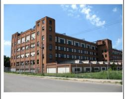
Large rectilinear 5-story brick clad steel framed industrial building with 6-story stair towers at each corner of the building and at center. Contains several intact industrial metal sash windows and many replacement windows which complement the scale and design of the originals. 1-story portion at north features saw-tooth skylights for additional interior lights. South elevation features 1-story portion and large metal silo.
